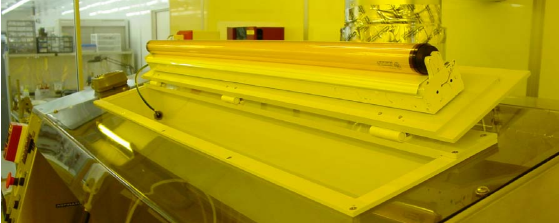
Figure 5. Changing hood lamp. Note the yellow filter to prevent unintended exposure of optical photoresist.
