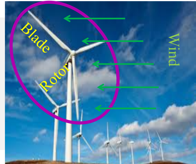
Horizontal rotational axis (traditional) wind turbine. 70-100 metre tall; 80-100 metre of blade diameter.
