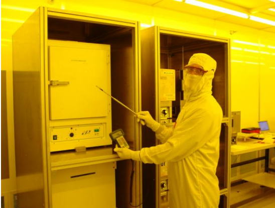
Figure 2. Hot-wire anemometer airflow measurement
