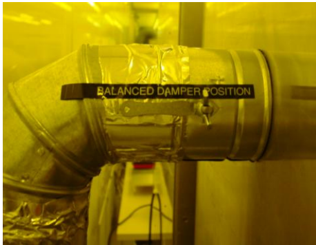
Figure 4. Upper left oven damper pos. Figure 5. Lower left oven damper pos.
