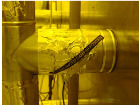
Figure 4. Upper left oven damper pos. Figure 5. Lower left oven damper pos.
