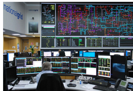
Fig. 1. User interfaces for power grid operators facilitate situation awareness, by providing information from which the power grid operator can estimate the state and predict its evolution. The sheer volume of information warrants the use of constructive tools (as opposed to ad hoc guidelines) to synthesize the information content of the interface. Image licensed under CC BY-ND 2.0.
