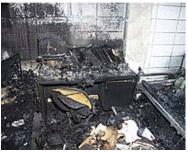
These post-fire photographs of the dorm rooms show the difference a sprinkler makes. There is little visible damage the in the top photo that had a sprinkler in the room; there was no sprinkler in the dorm room in the lower picture.
